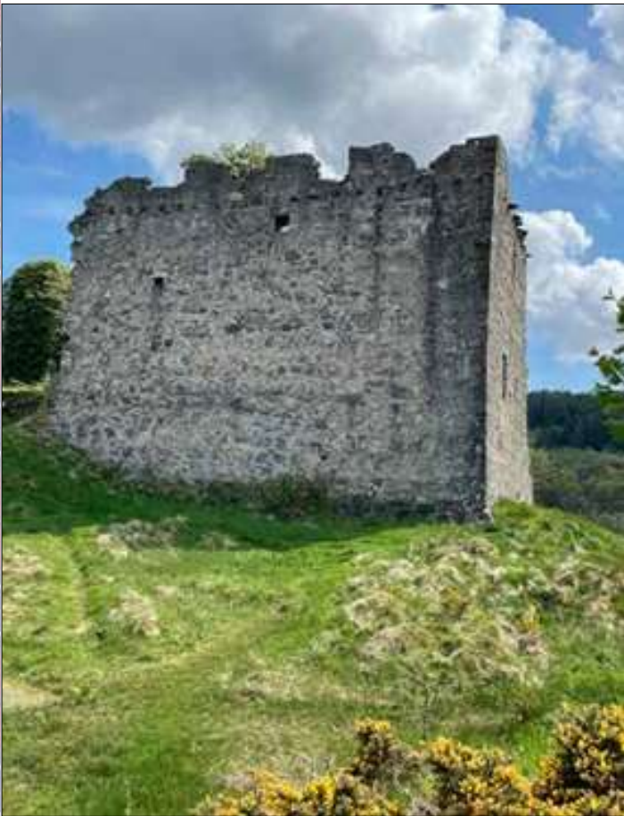
This face of Old Castle Lachlan has been cleared of the ivy that both held the ancient stones together while forcing them apart. Clearing the ivy is an important first step in Clan Maclachlan Society's plan to preserve this historic ruin. Photo: Cyndi Boman.
